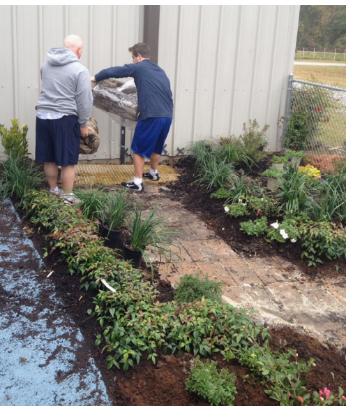
Installation of the water feature for the garden.
