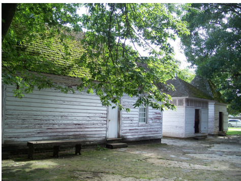
▲ Outbuildings and a kitchen garden are located behind Wetherburn's Tavern.
